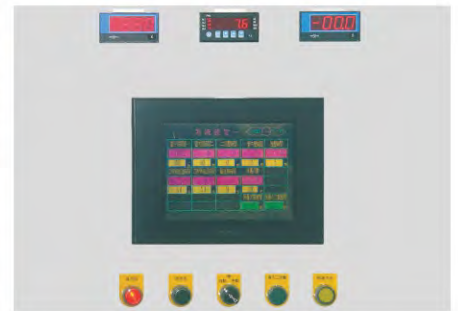
Touch Screen Human Machine Interface : Easy to understand & operate.
